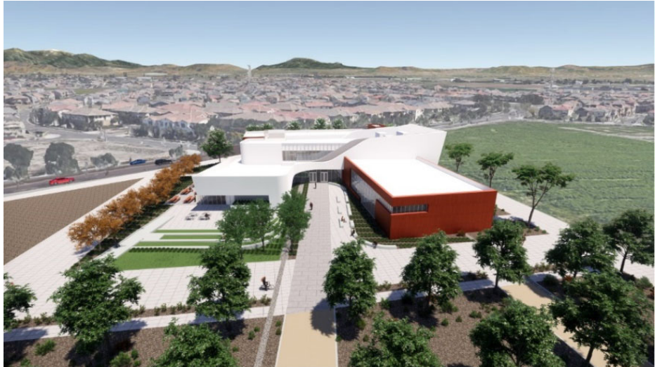
CHINO IB Building View
