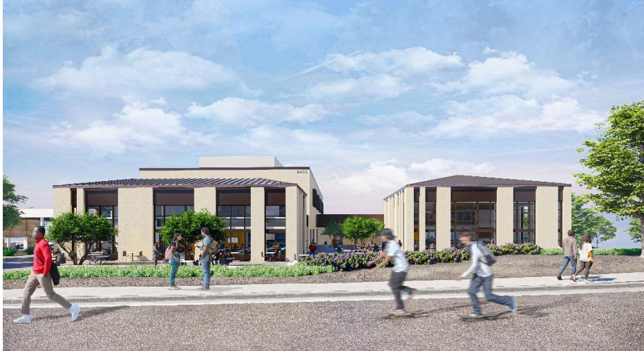
RANCHO CUCAMONGA MACC Renovation & Addition
